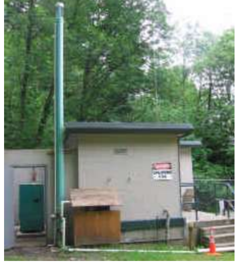
FIGURE 6 Aeration Tower for Corrosion Control Pilot Test
