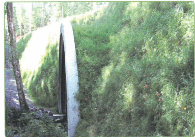
10m (33ft) tall municipal roadway
