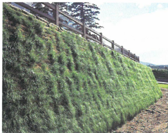
5m (16ft) tall landscape retaining wall
