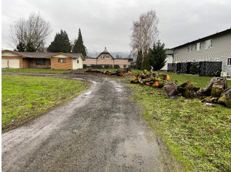
Figure 2: Existing conditions at the subject site, image collected January 11th, 2021.
