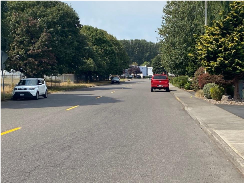
Looking West Along Mitchell Avenue from Proposed Site Access
