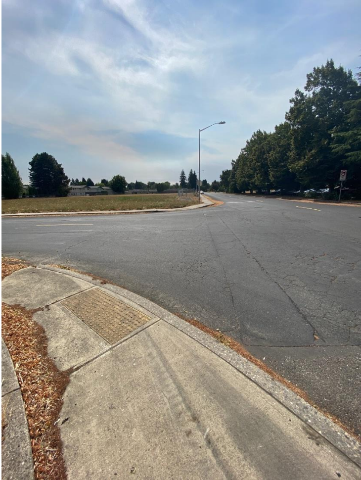
Adjacent Columbia Street/Glenwood Street Intersection
