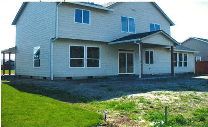
REAR VIEW (NORTH) 04-18-13
