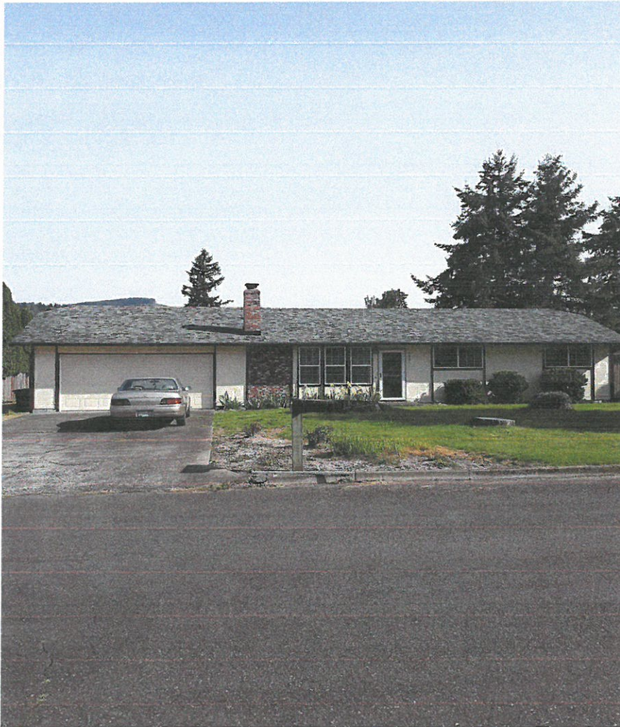
4/25/2019-2081 Spruce Ave, Woodland, WA 98674- Street view
