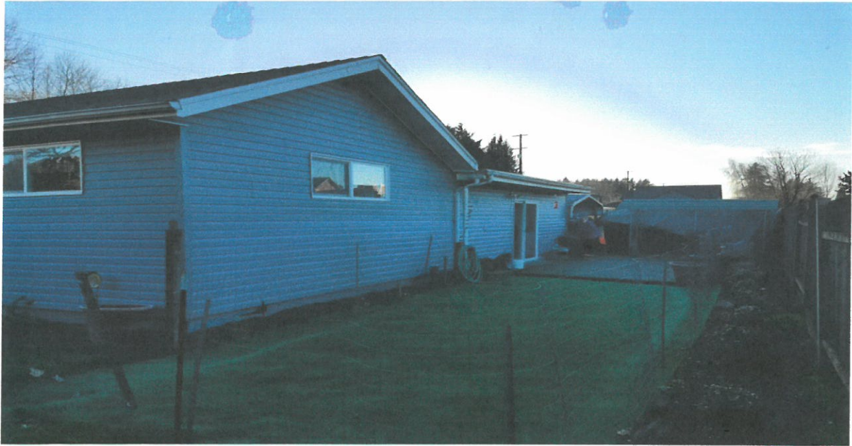
Photo One Caption: Picture shows Back of house, looking Southwesterly. Photo taken 12/20/2017.
