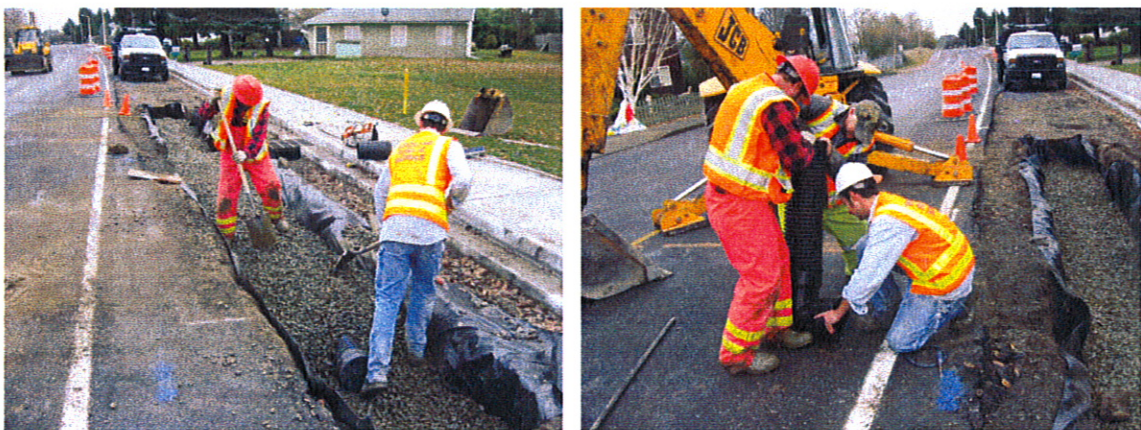
2011 Sidewalk Project South Pekin Road Catch Basin Installation
