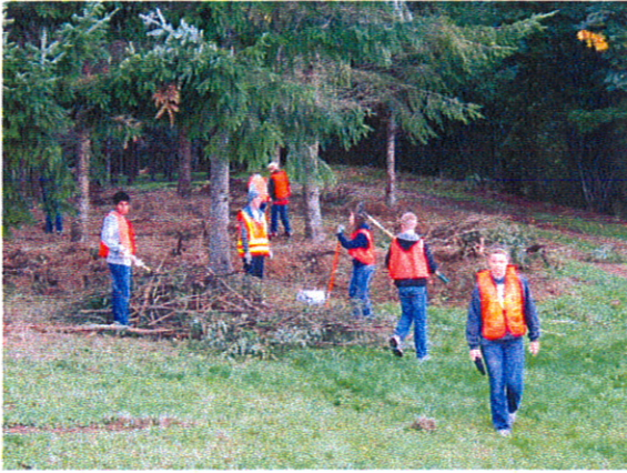
WWTP - Tree Clearing
