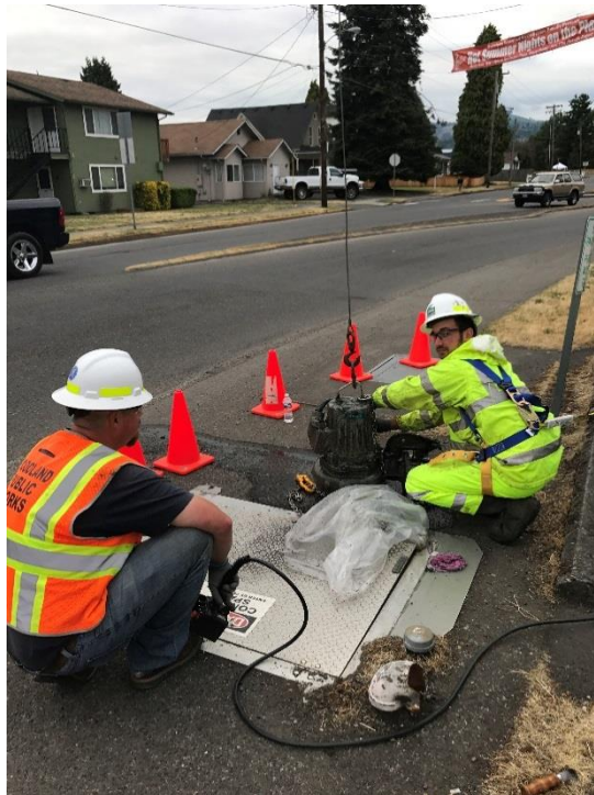
SCOTT SUMMERS & TYLER LEE PULLING PUMP ON LIFT STATION #2
