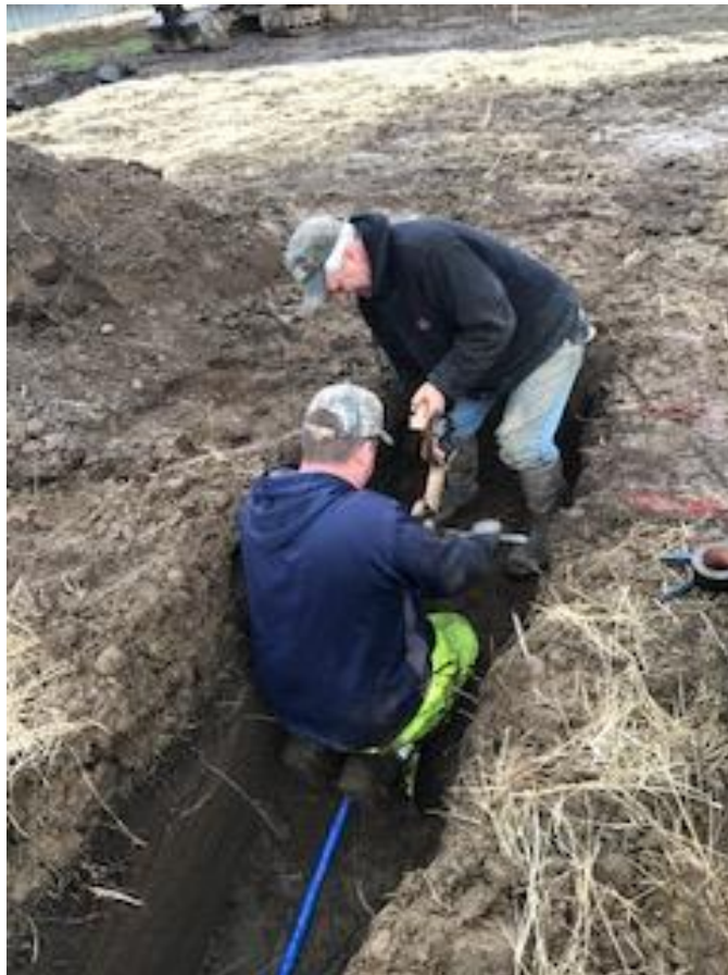
CREW WORKING ON NEW WATER TAP ON GUN CLUB ROAD
