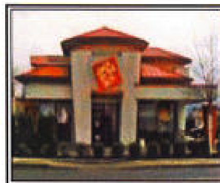
Figure 19 Good example of articulation and massing
