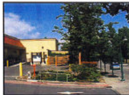
Figure 61 Loading area screened by fence and landscaping
