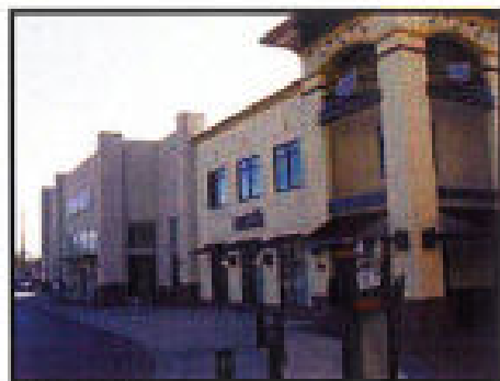
Figure 18 Good example of horizontal and vertical offsets
